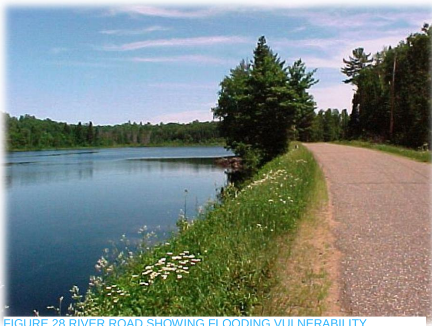
FIGURE 28 RIVER ROAD SHOWING FLOODING VULNERABILITY
