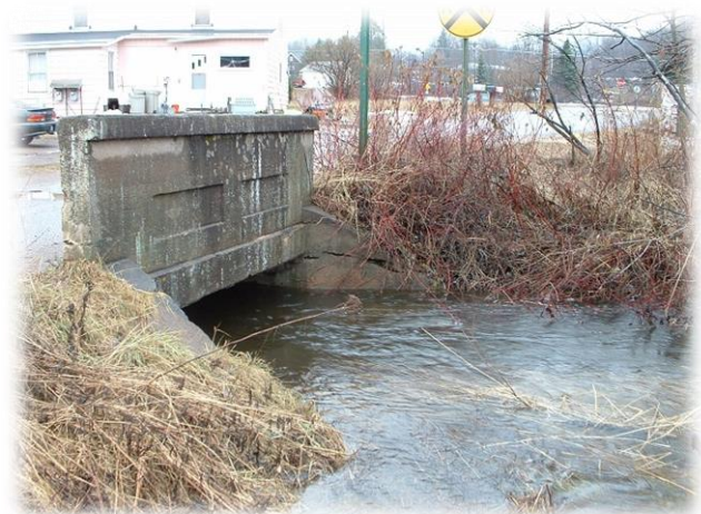
FIGURE 30 COUNTY RD PCC BRIDGE OVER ELY CREEK
