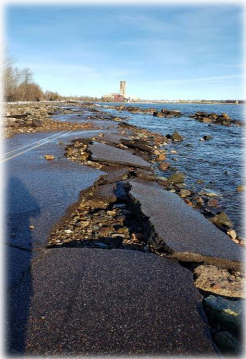
FIGURE 7 SHORELINE EROSION ON LAKESHORE BLVD IN MARQUETTE
