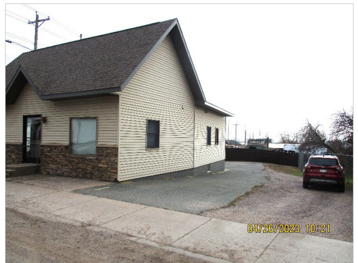
Oblique view of the building, looking north-northeast from Division St.
