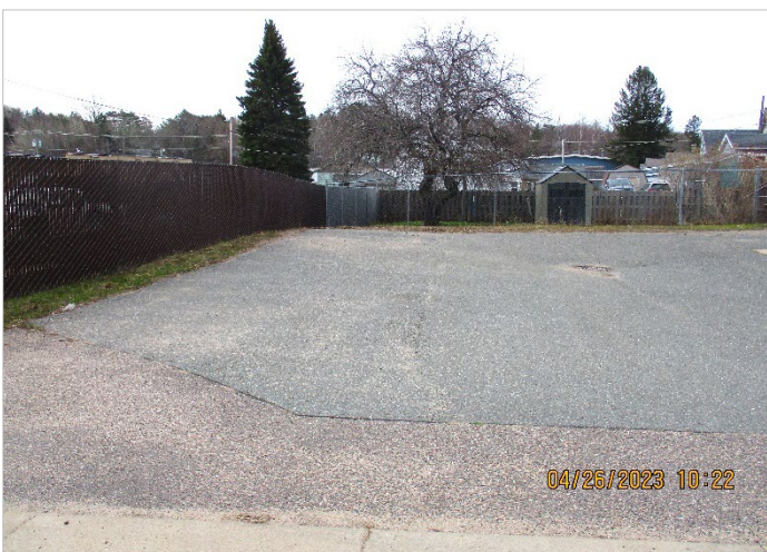
The parking lot to the rear of the building, on the east side of the lot.
