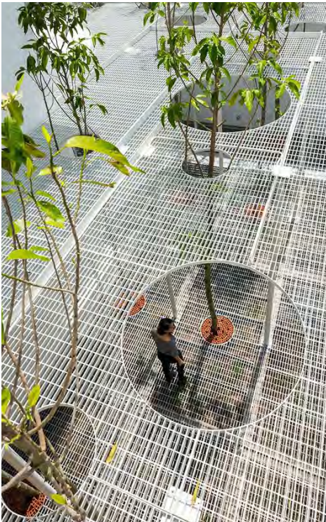
Buildings 3 zone: Metal grading deck
