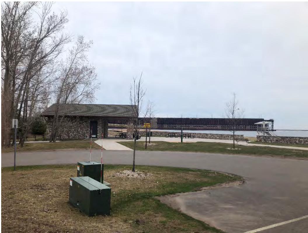
Photo 14. Clark Lambros Beach Park restroom facility and parking area (constructed in 2015).
