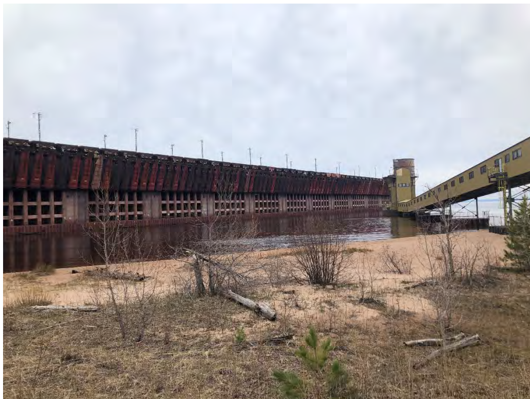
Photo 17. Looking northeast at the Marquette Ore Dock and coal unloading structure.
