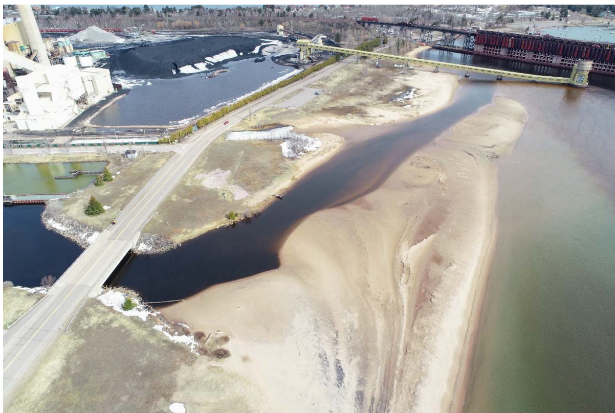
Photo 4. Aerial photo looking north at the sediment plume encroaching on the Marquette Ore Dock.
