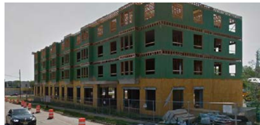
Lofts on Louis Construction (now complete), Jackson, Michigan (image: Google Street View)
