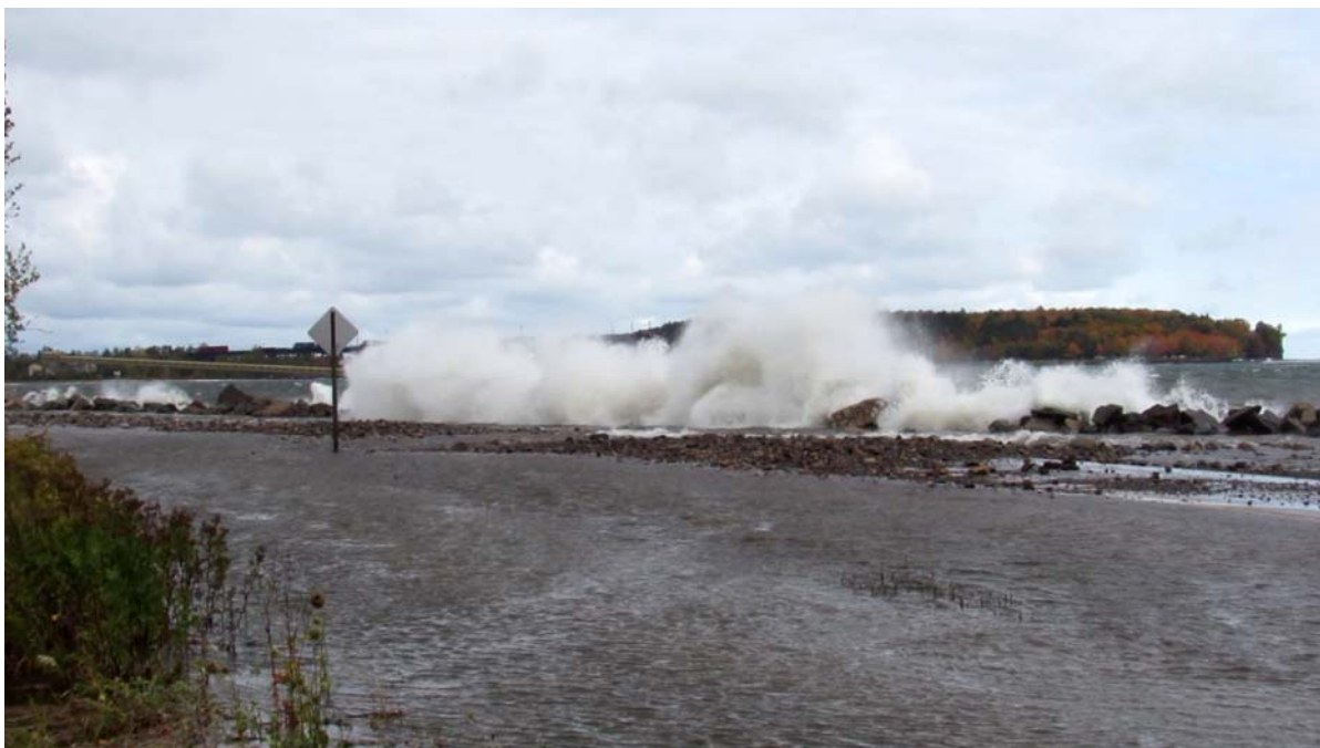
Photo 1. Looking north at the Port access road (Lakeshore Boulevard) during a storm.
