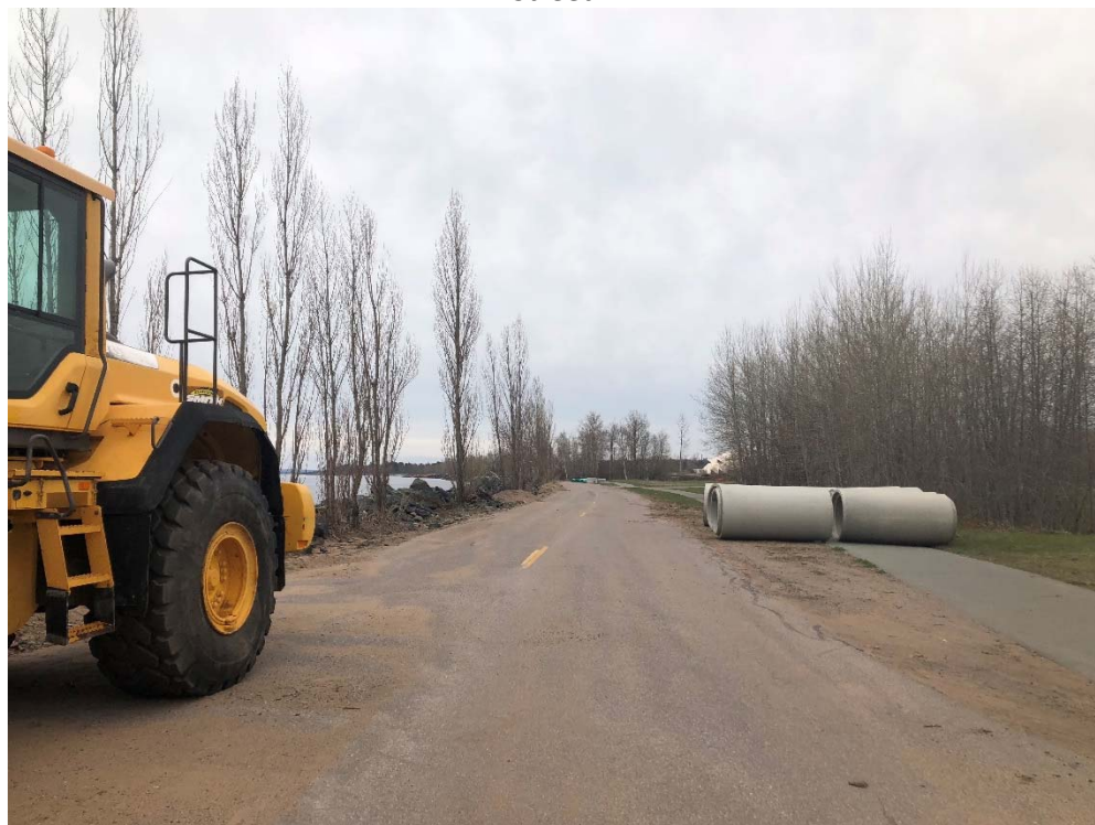
Photo 10. Looking south at Lakeshore Boulevard from the intersection with Hawley Street.
