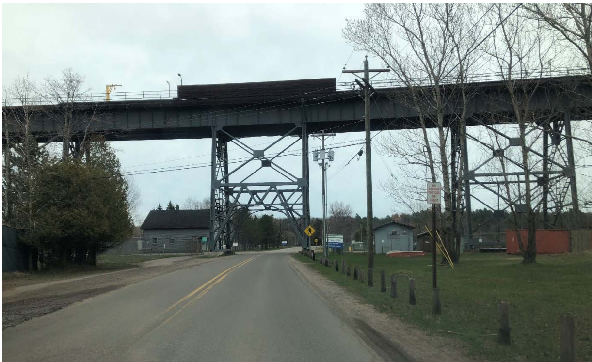
Photo 19. Looking north at the LS&I dock facilities and outbuildings (first construction in 1911).
