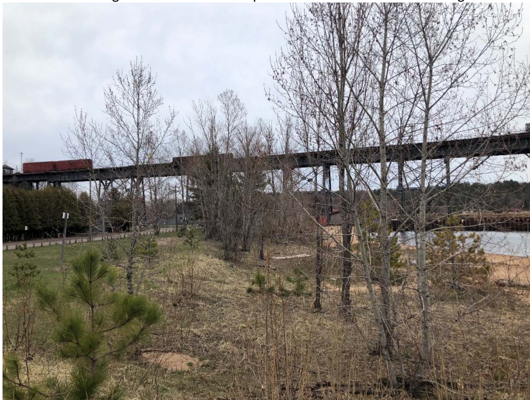
Photo 18. Looking north at the natural shoreline adjacent to the Marquette Ore Dock.
