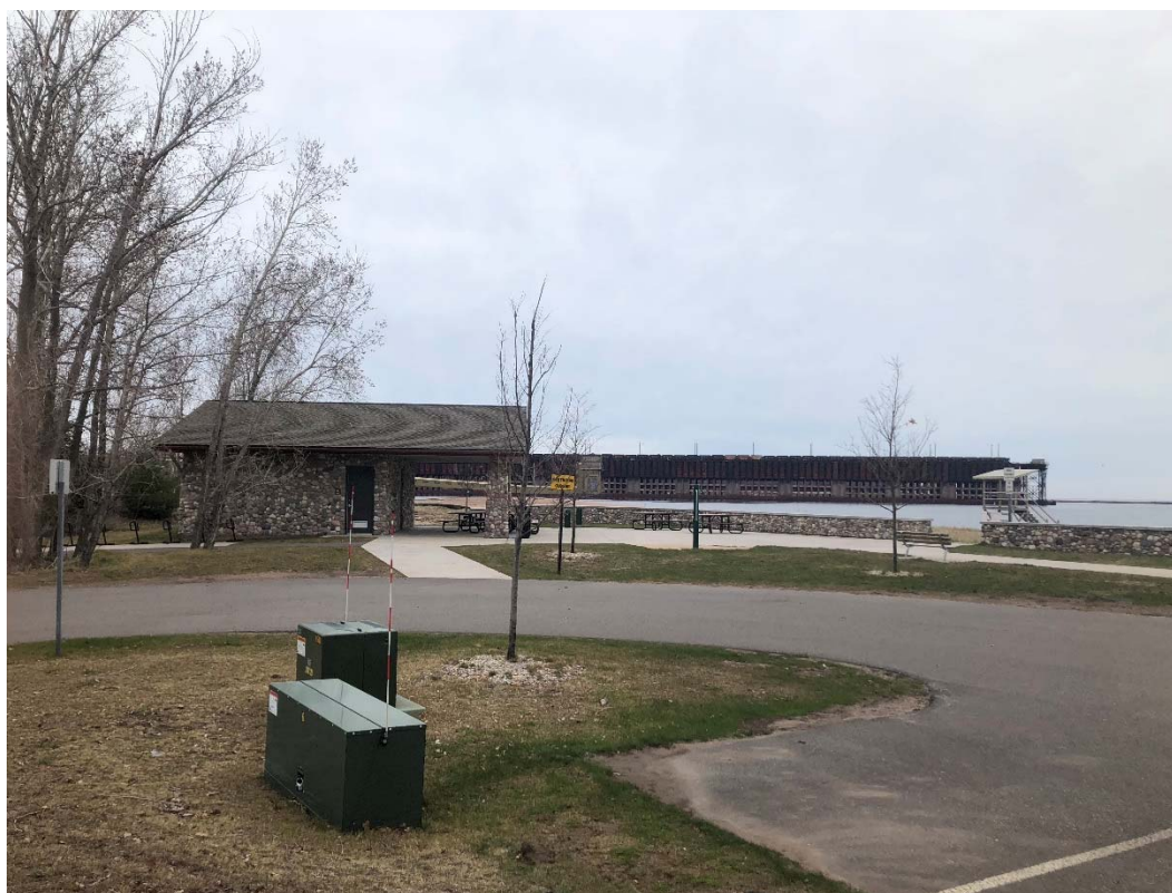
Photo 14. Clark Lambros Beach Park restroom facility and parking area (constructed in 2015).
