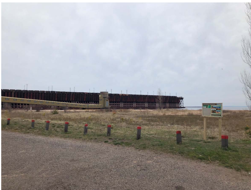
Photo 16. Looking northeast at natural beach and parking area adjacent to the Marquette Ore Dock.
