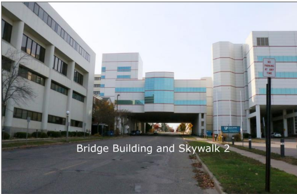
Figure 7. Bridge Building, view to the west
