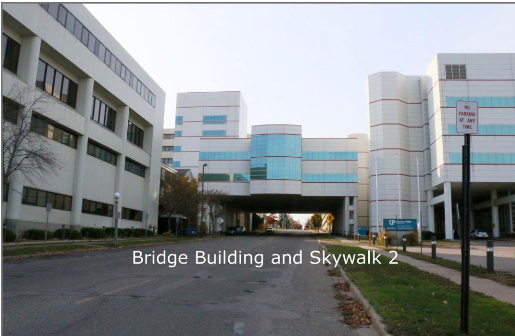
Figure 5. Bridge Building, view to the west
