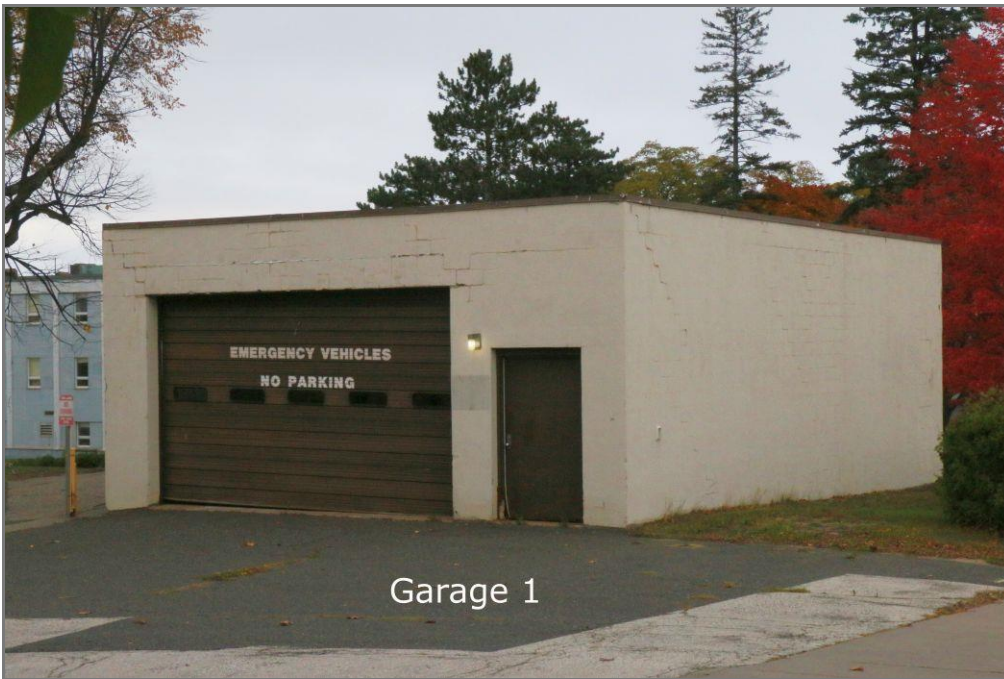
Figure 13. Garage, view to the northeast
