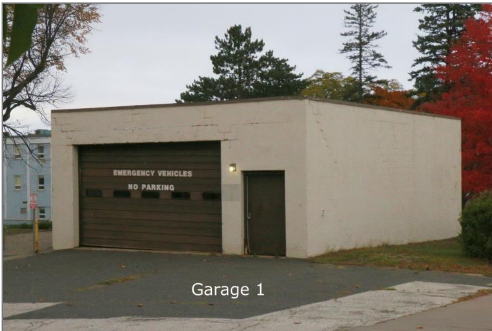
Figure 15. Garage, view to the northeast
